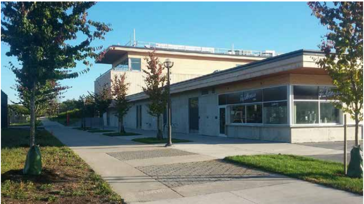
Photo 4 – Exterior View of Field House
