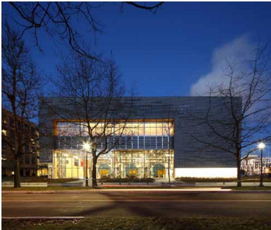
Photo 2 – Exterior View of Entrance
