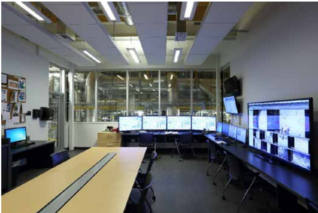
Photo 6 – Interior View of Controls Room
