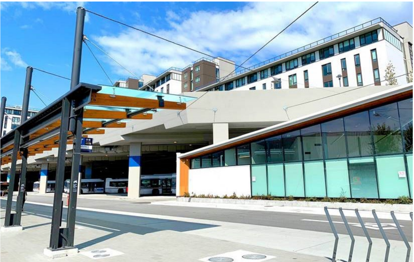
Photo 2 – View from South Passenger Pick-up Zone looking towards Layover and Drivers' Facility, with Exchange Residence over
