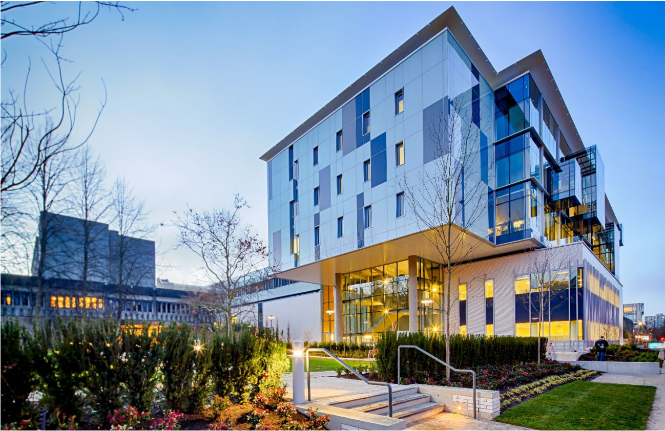
Photo 3 – Exterior View South Side
