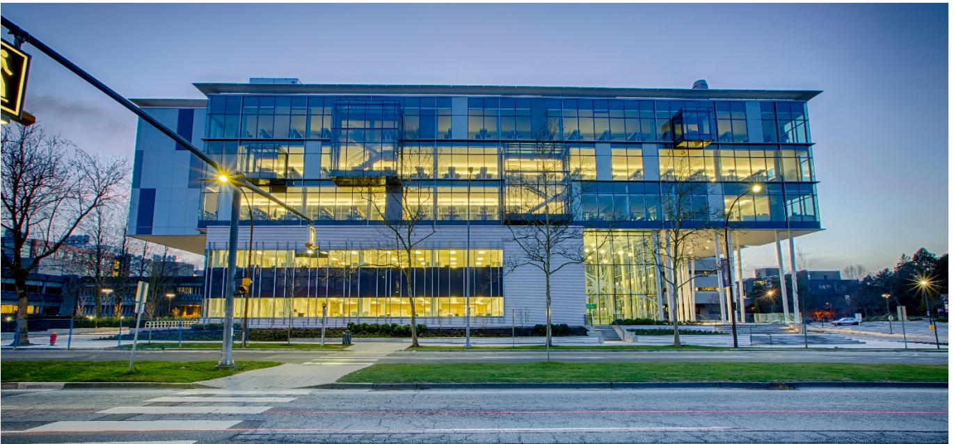
Photo 2 – Exterior View from Wesbrook Mall
