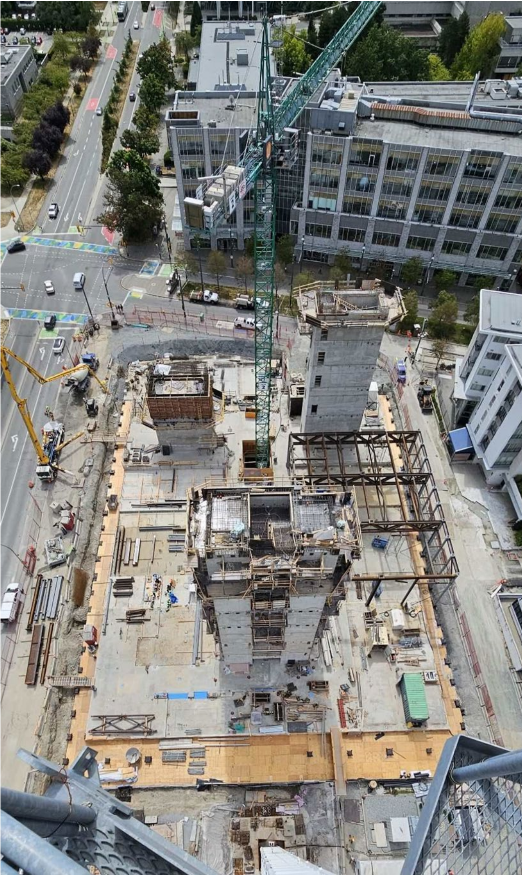
View from above showing elevator cores
