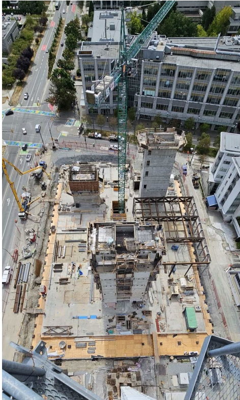
View from above showing elevator cores
