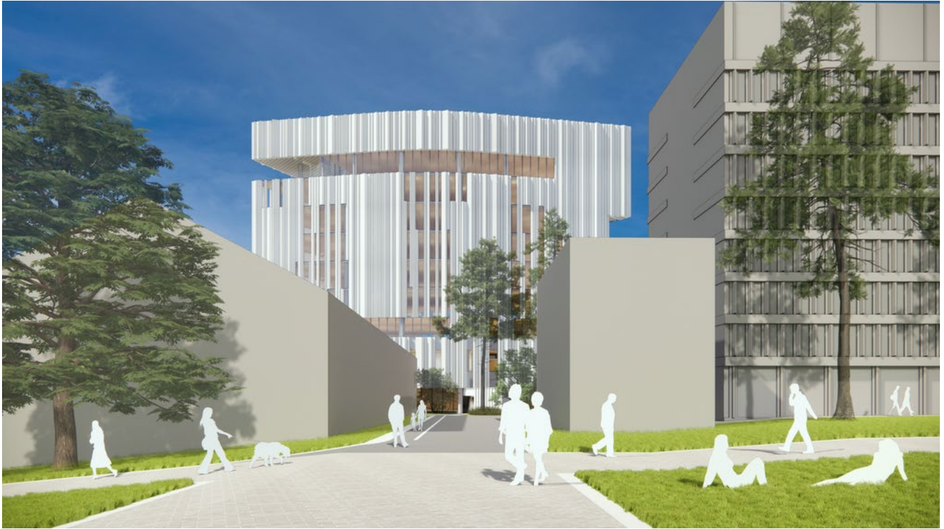
Street view across University Boulevard facing north-west
