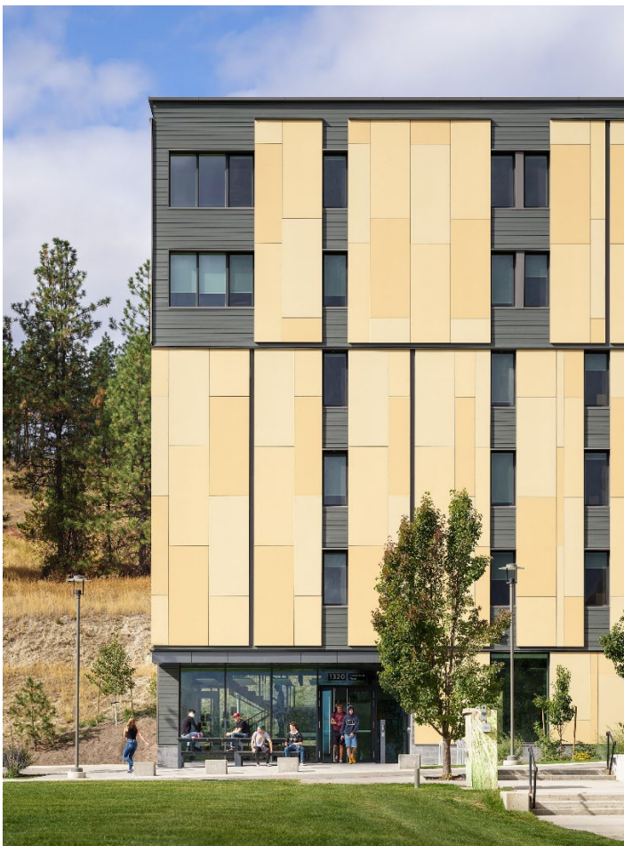
Photo 2 – Exterior View – Entrance from Purcell Photo Courtesy of UBC Properties Trust
