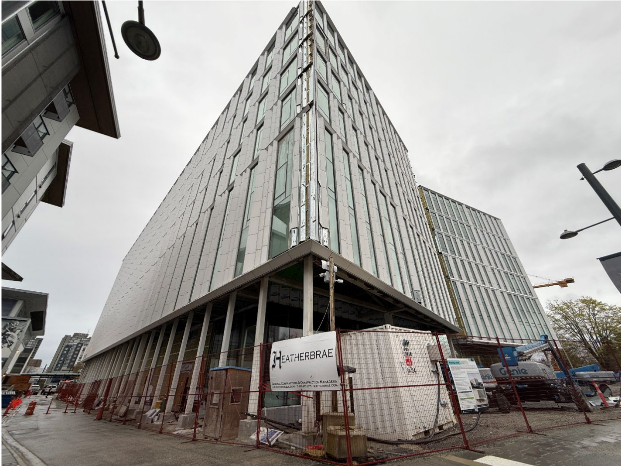
Recent Construction Progress Photo (April 2025): View from University Boulevard (south-west corner)
